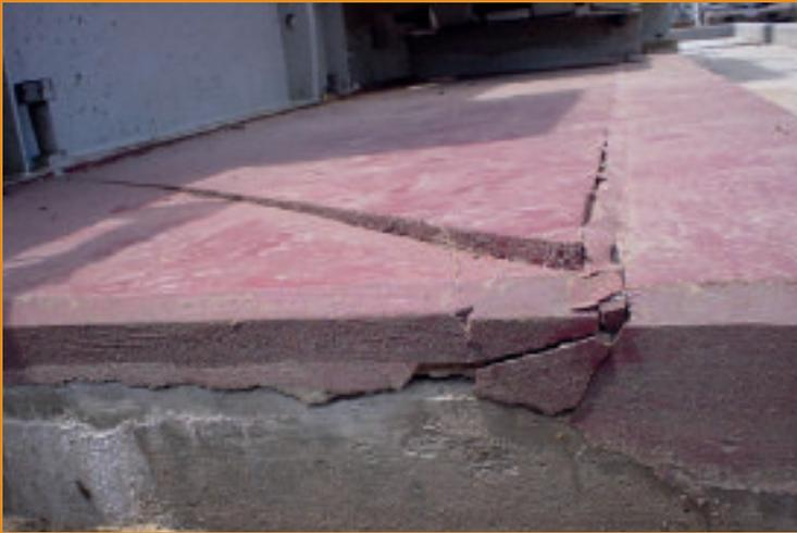
**Grout cracking and edge lifting due to excessive grout placement, lack of expansion**
