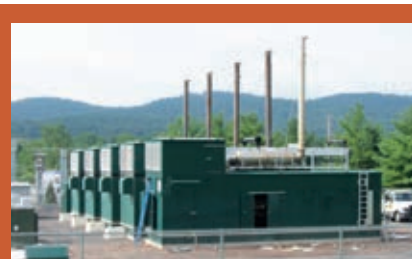
Engines powered by unconventional sources of gas, such as these using landfill gas, are being developed quickly in many markets. As engine manufacturers adapt their engines to run on different fuel types, one area of concern is the increased stress on engine oil.
