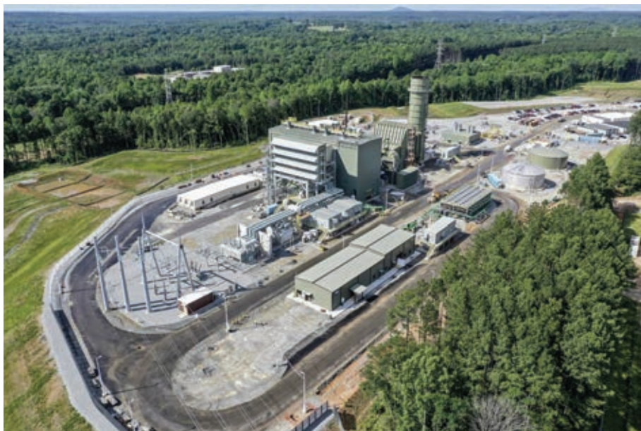
The validation of the HL-class gas turbines is taking place in real-life conditions at the Lincoln County, North Carolina, USA, where one SGT6-9000HL is connected to the grid during a four-year test process.
